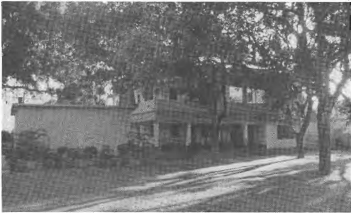
The Hostel Building That Now Houses 35 Children. It Is A Two Story Building Constructed of Concrete With Porches On Each Floor That Extend Completely Around The Living Area.
