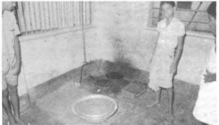
This Is A Cooking Area In Addition To The Above One. This Is A Gas Burner. The Gas Is Supplied From A Reservoir To The Rear Of The Hostel. The Gas Is Formed Through A Process Of Animal Dung And Water.
