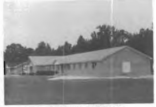
Grace Facilities With New Addition And Parsonage
