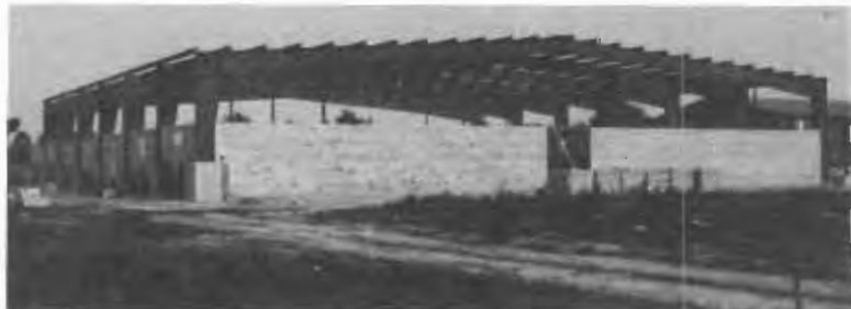
New Facilities For FFWB, Florence
