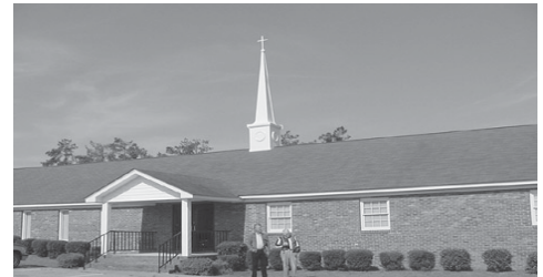
Liberty FWB Church and Pastor Roger Tripp celebrated Easter with a brand new steeple that they installed on the Church on Good Friday.
